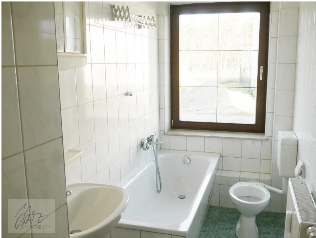
Erdgeschoss links - Badezimmer
